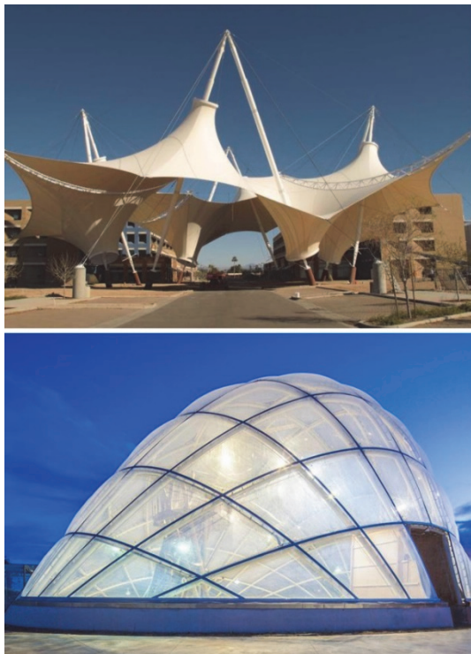
Figure 1 Membrane structures with negative (top, photo credit: FTL Studio) and positive Gaussian curvature (bottom, photo credit: Quintin Lake)
