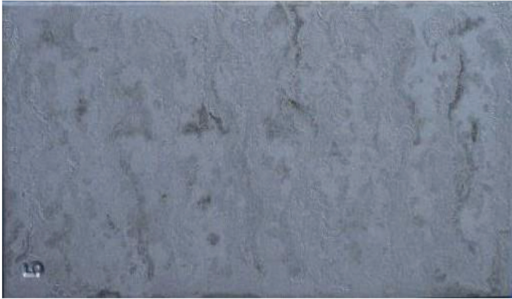
Fig. 4 Example of sample surface after corrosion test and cleaning [14], [21]
