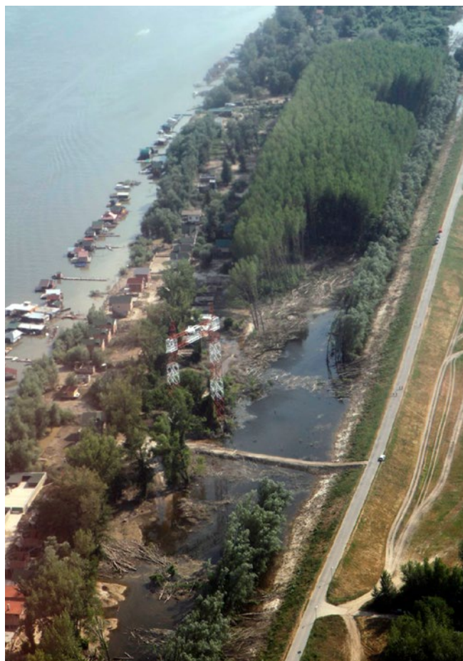
Picture 4 – drone photo of the illegal construction buildings in the flood defense area of the River Sava Embankment, provided by the organization "Savski Nasip" (April 7, 2021 - F.B. and internet page).
