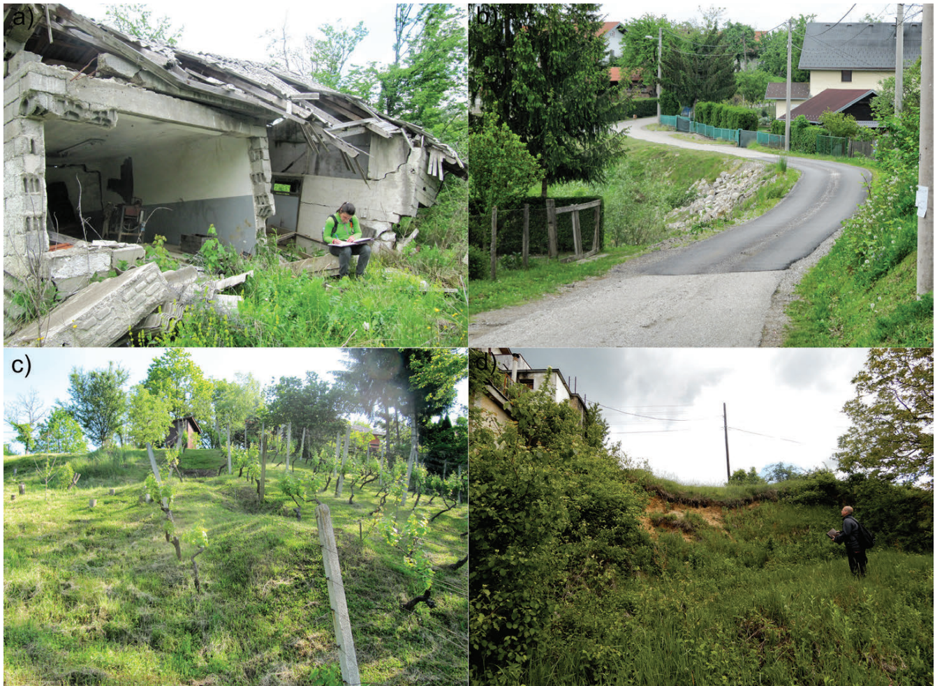
Figure 2. Landslide damage in the Kravarsko area: a) destroyed storage in landslide body; b) road mitigated by rock embankment and “fresh” asphalt; c) damaged vineyard in the main body of a landslide; d) landslide main scarp by a house (photos by HGI-CGS, 2019).
