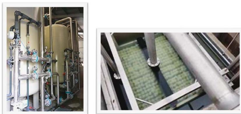
Fig 9 Waste water purification with ion exchange resin and membrane bioreactor (MBR) in Olimpias Tekstil d.o.o. [36]
