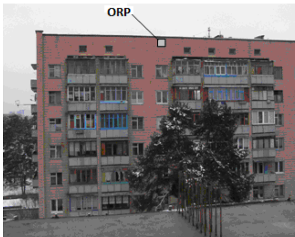
Fig. 6. Location of ORP 1 in the form of a retro reflective foil target on the facade of a high-rise building.
