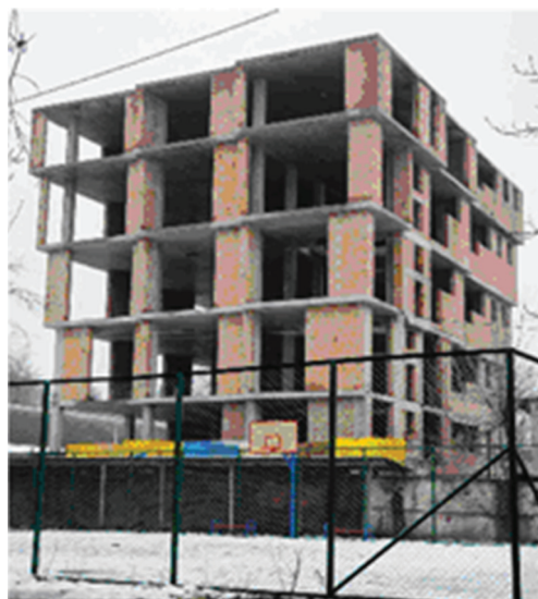
Fig. 4. View of a high-rise building constructed in a monolithic frame way.
