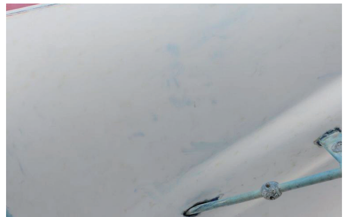
Figure 9. The sane hull surface after grinding the antifouling paint and protective epoxy primer
