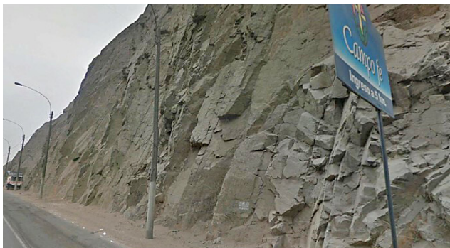
Figure 3: View of rock mass 1
