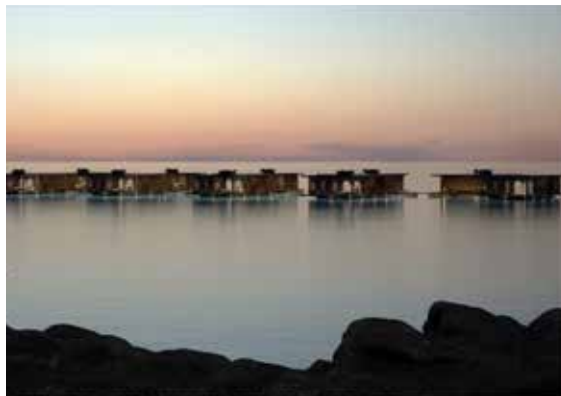
Figure 3. Floating houses resort
