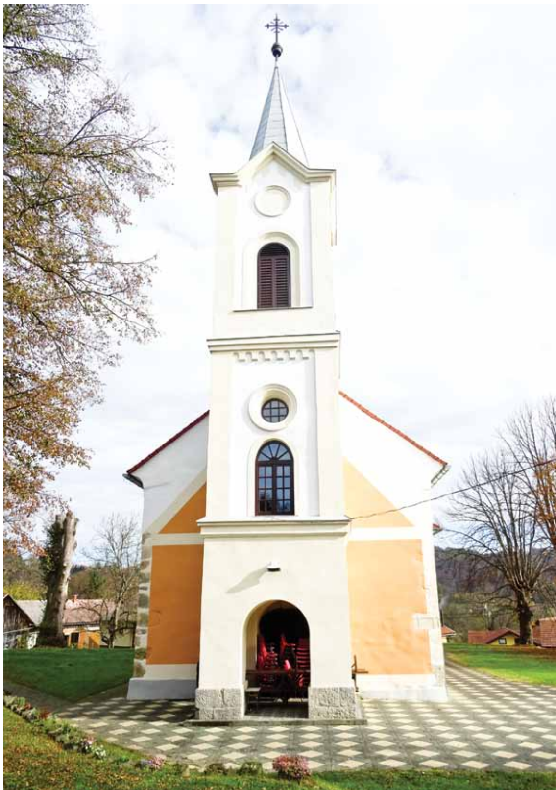
Sl. 5. Crkva Uznesenja Blažene Djevice Marije u Novigradu na Dobri s urnom uzidanom na pročelju (snimio: L. Čučković) / Fig. 5. Church of the Assumption of the Blessed Virgin Mary in Novigrad na Dobri with the urn walled in its façade (photo: L. Čučković)
