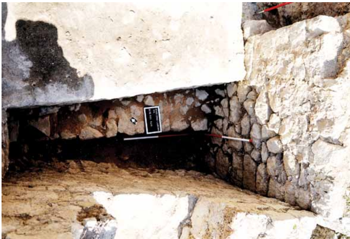
Sl. 10. Pogled na zid 14, ispod zida 13 (snimio: M. Rašić) / Fig. 10. View of the Wall 14 under the Wall 13 (photo by M. Rašić)
