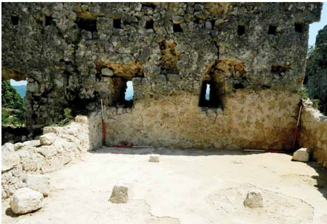
Sl. 13. Prostor sonde OHB-1 s podnicom i ugrađenim bazama (snimila: E. Vučić) / Fig. 13. The area of the probe OHB-1 with plaster pavement floor and inlaid pillar bases (photo by E. Vučić)
