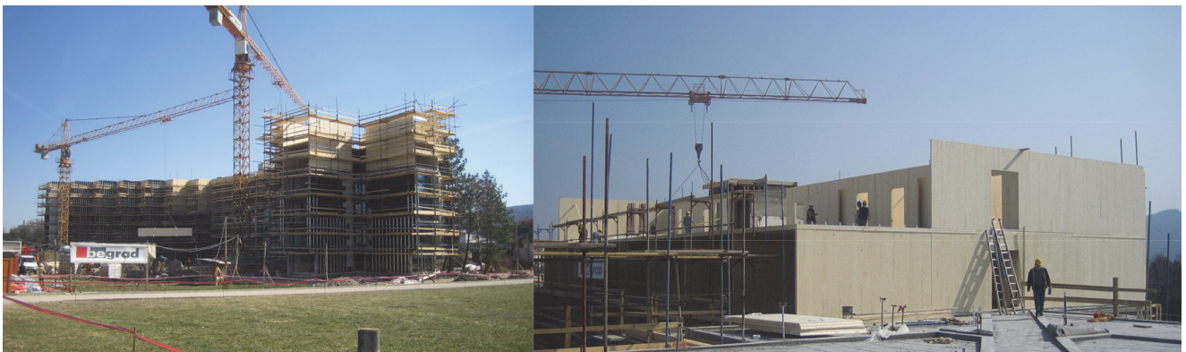
Figure 16. Assembly of Xlam structure
