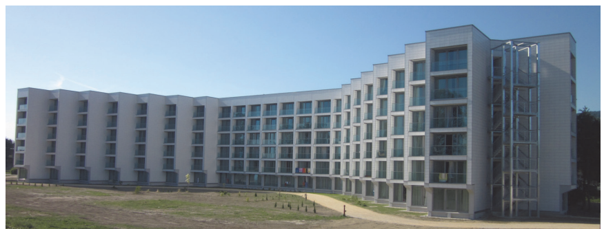
Figure 17. Finished hotel with two-storey upgrade
