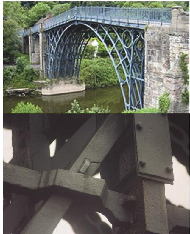
Figure 8 The Iron Bridge (top), and cracked supports (bottom), [29]
