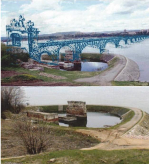
Figure 6 Trajan's bridge schematic presentation (top), remains of stone pier (bottom)
