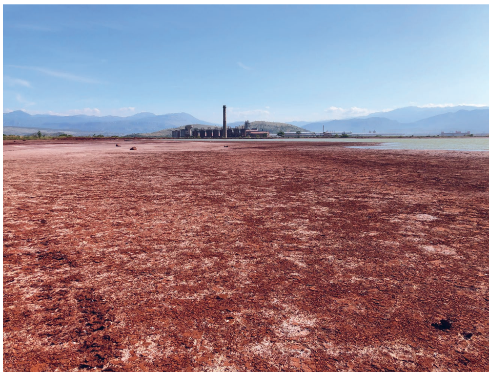
Figure 7. Red mud - bauxite residue tailings dams, Podgorica.
