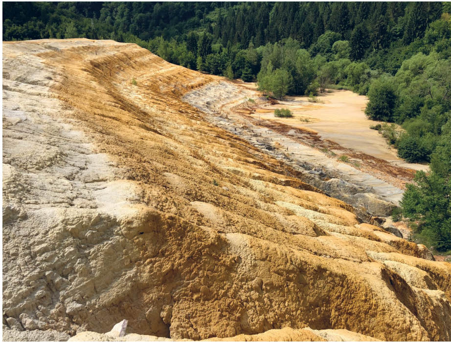
Figure 8. Flotation tailings dam at "Gradac".
