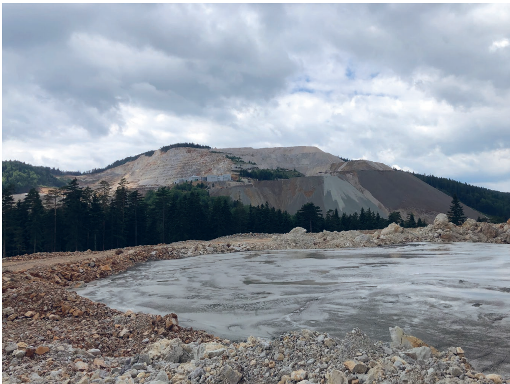
Figure 4. The lead and zinc mine at “Šuplja stijena”, Pljevlja. Open pit, waste rock dump and flotation tailings.
