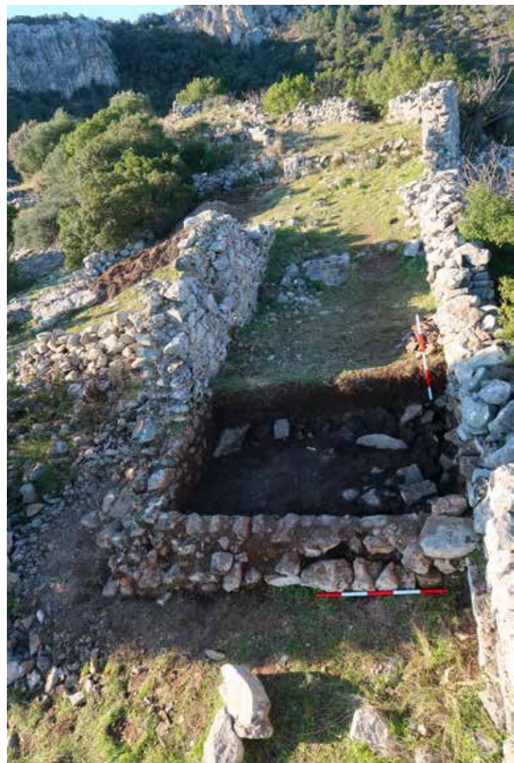
Sl. 6. Sonda I, dio sjeverozapadnog bedema i ostatci prostorija koje su se pružale uz njega. Fig. 6 Test Pit I, a part of the north-west rampart, and the remains of rooms that stretched along it.
