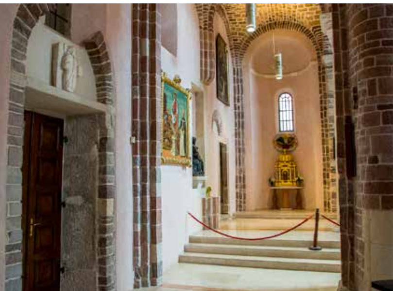
Sl. 11. Sjeverni brod katedrale s arheološkim prikazom starijih vrata koja su bila blokirana tijekom dovršetka katedrale prije 1331. (izvor: Zbirka D. Mergela) Fig. 11 North nave of the Cathedral with the archeological presentation of earlier doors which were blocked during the completion of the Cathedral before 1331. (source: collection of D. Mergel)
