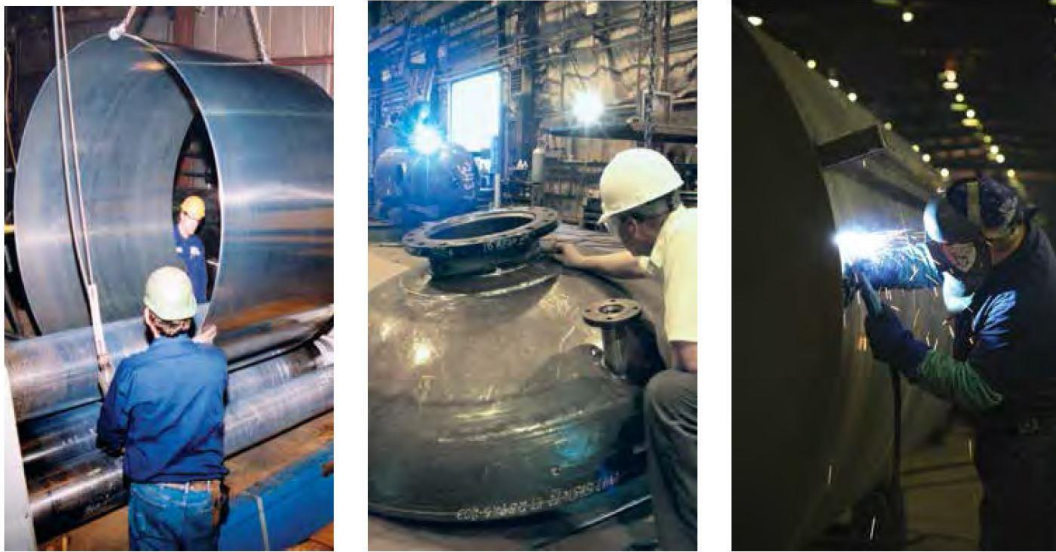
Figure 1. Forming and welding of a pressure vessel.
