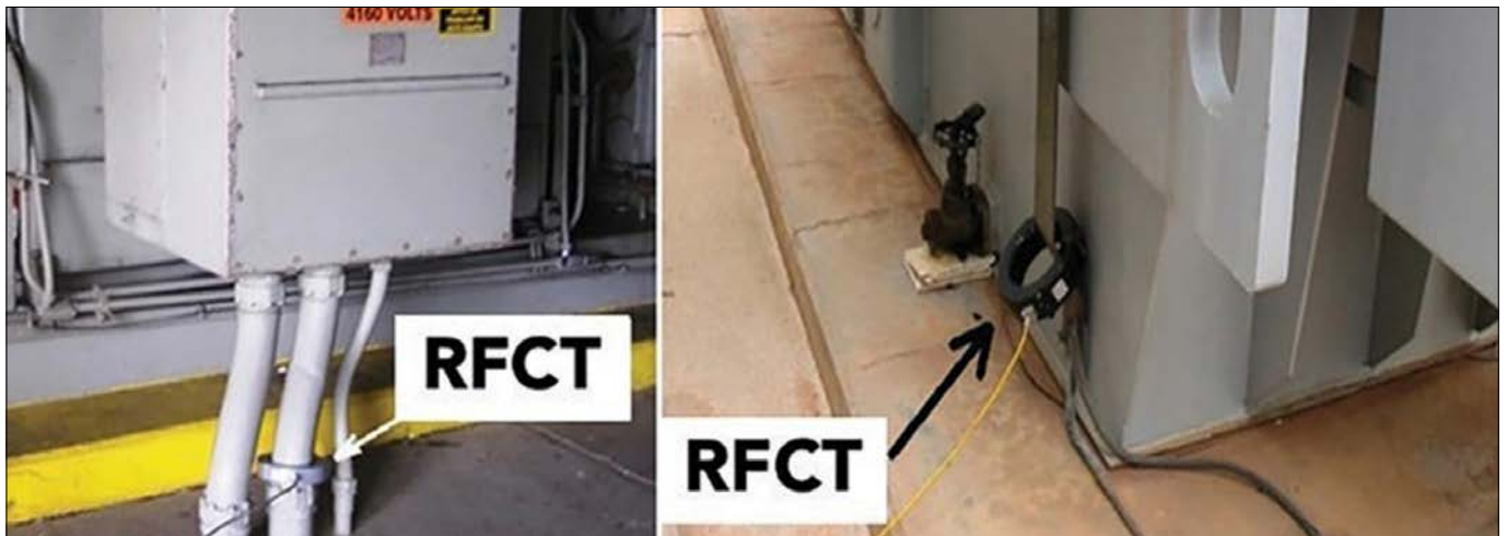
Figure B: Radio Frequency Current Transformer (RFCT)
