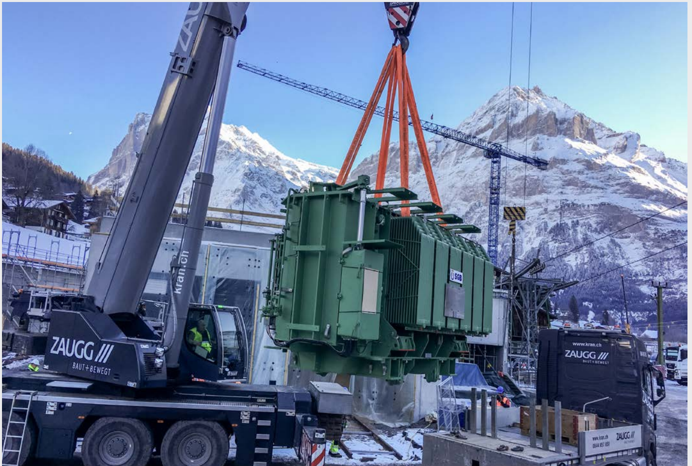
Figure 2. Installation of 25 MVA transformer in Grindelwald, Switzerland (photo BKW, Switzerland)
