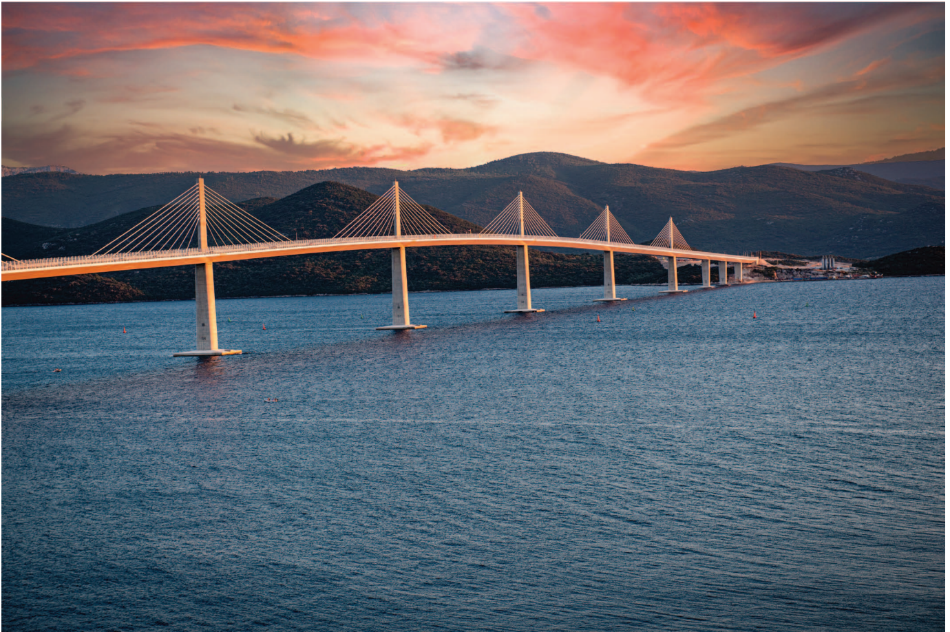
Figure 1 View of the construction of the Pelješac bridge
