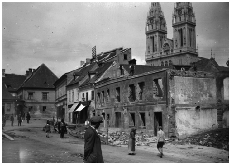
Figure 4: Changes in the city. Dolac before being demolished. (GMNG-FKD. Photography collection, 6329)
