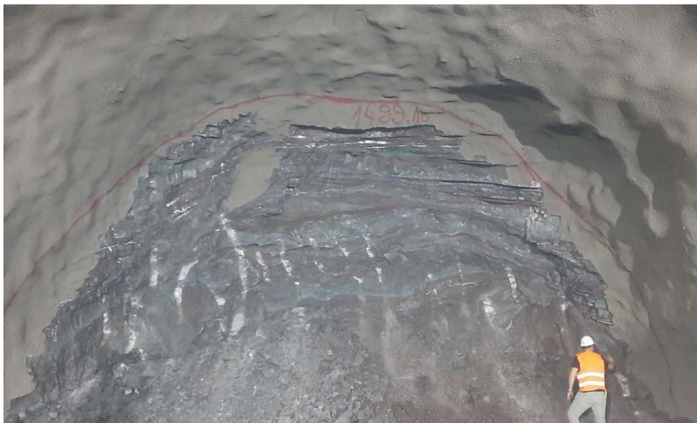
Figure 2. View of the work face, chainage 1+499.10 - left tunnel tube
