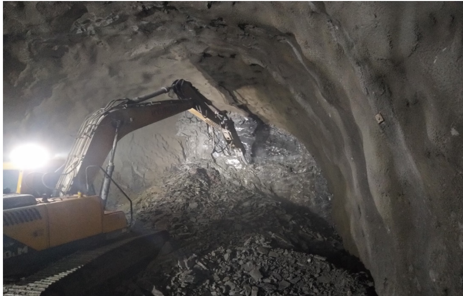
Figure 6. Machine excavation of full cross section in LTT at chainage 1+518.00 to 1+520
