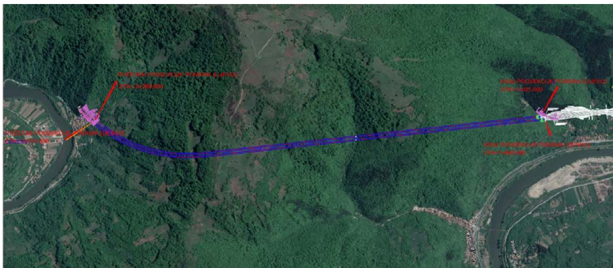
Figure 1. Geographical position of the Zenica tunnel on the Corridor Vc route
