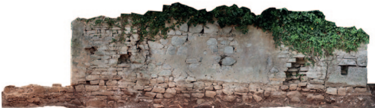
Fig. 2 Orthophoto of the rear wall of the Church of the Holy Cross and a segment of the earlier wall (photo and processing by: K. Bartolić Sirotić) Sl. 2 Ortofoto snimak začelja crkve sv. Križa i segment ranije arhitekture (snimila i obradila: K. Bartolić Sirotić)
