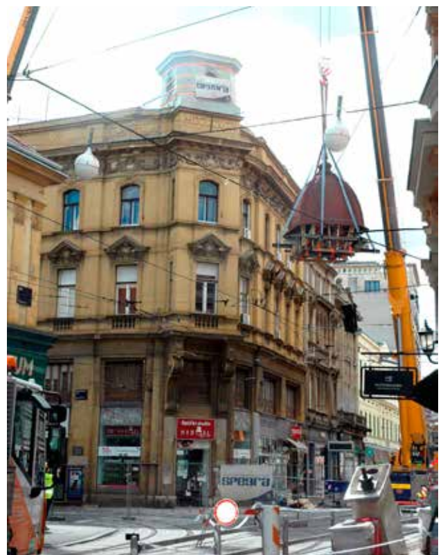
17 Demontaža kupole, 30. travnja 2020. (foto: P. Puhmajer) The demounting of the dome, 30 April 2020, (photo: P. Puhmajer)
