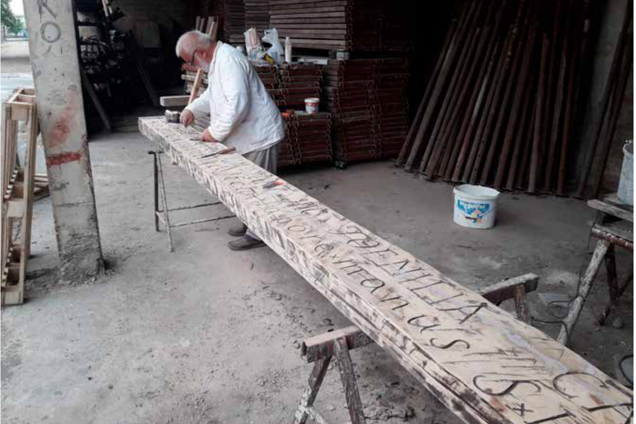
13 Obnova drvene grede (foto: M. Ožanić, 2018.) Restoration of the wooden beam (photo: M. Ožanić, 2018)
