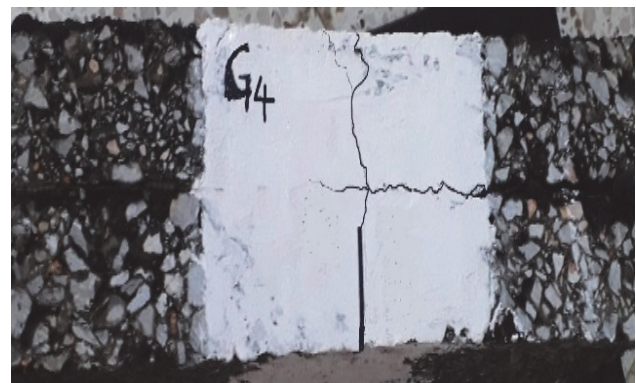
Figure 10 Crack propagation of the G4 geogrid (50 °C)
