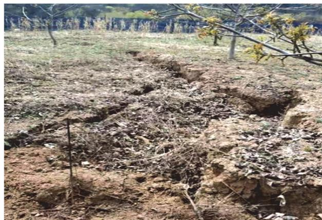
Figure 1 Residual deformation of the foundation of the mined-out areas
