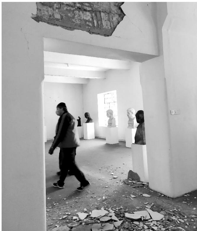
**Figure 4.** *Big cracks on the walls and ceilings in the interior*
