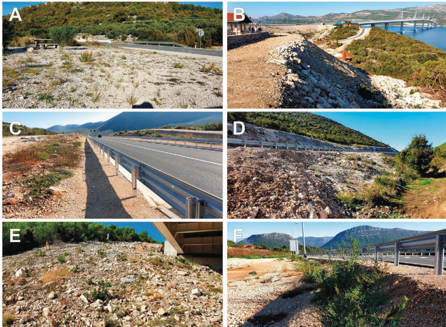
Fig. 2. Ruderal sites along the access roads to Pelješac Bridge in autumn 2022: above the village of Komarna on the mainland (A), near the villages of Brijesta (B), Dančanje (C) and Metohija (D), and above Prapatno Bay (E-F) on the Pelješac Peninsula (photo: N. Jasprica).
