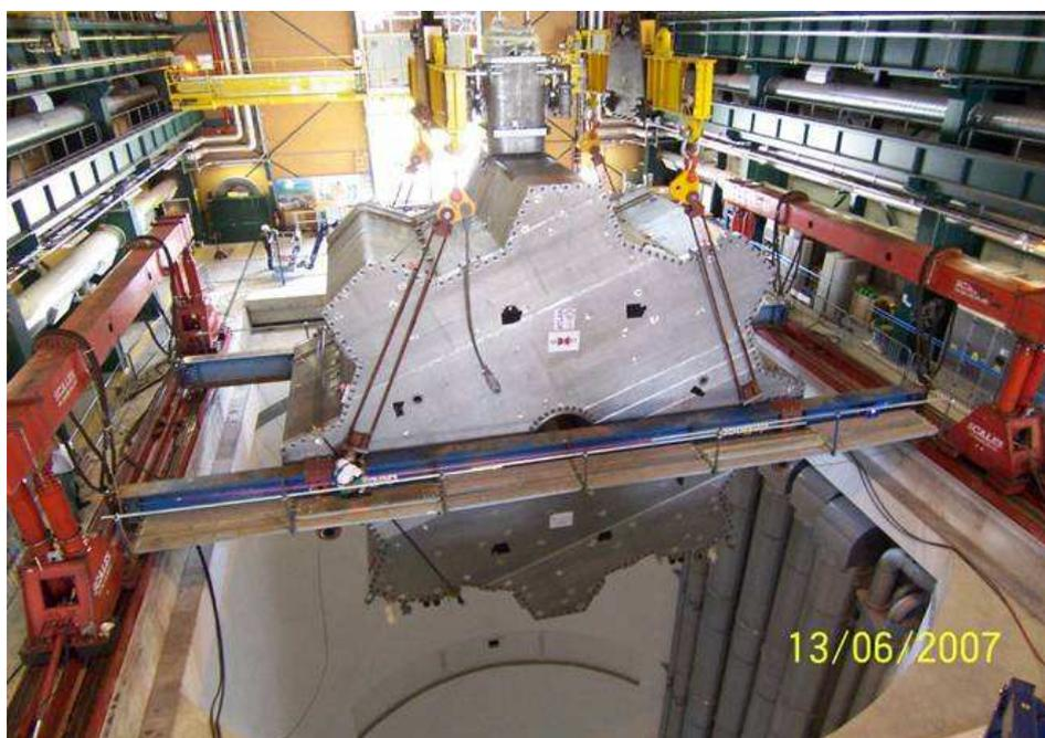
Fig. 1. One of the endcap toroid magnets being lowered into the ATLAS experimental cavern.
