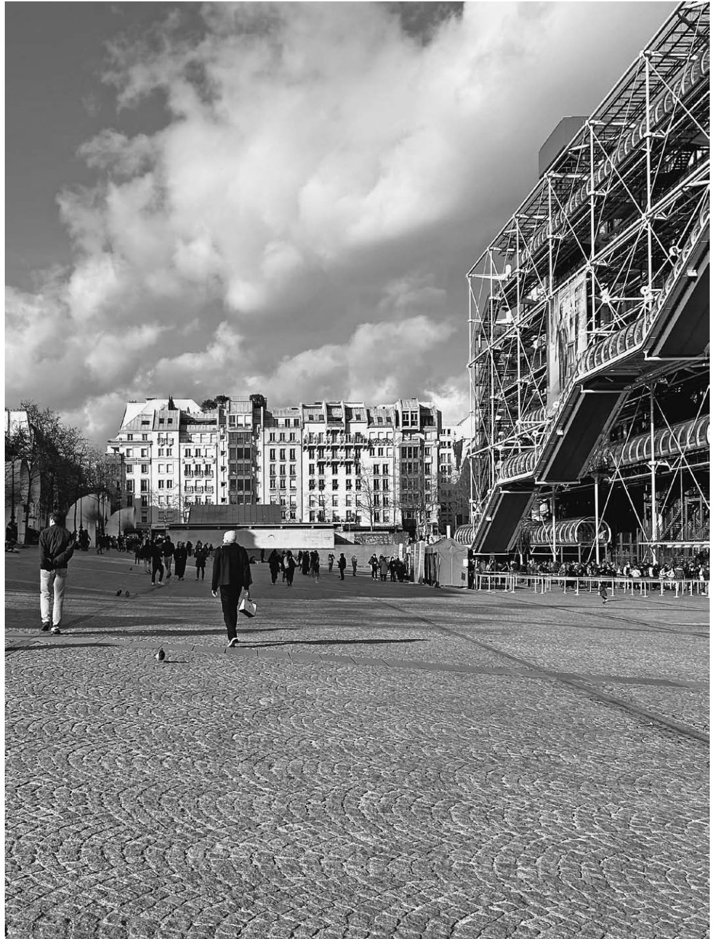
FIG. 1 CENTRE POMPIDOU, PARIS, FRANCE
