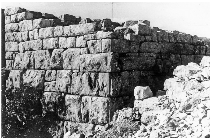
Fig. 14. View on the E and the N walls of Tor after the bombing by the Italian occupying forces in 1943. Photo from Nov. 24th 1947 by Niko Duboković-Nadalini. Courtesy of AMS.
