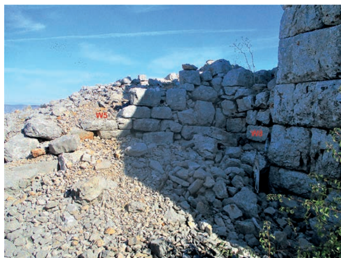
Fig. 21. View from S on the W wall of the tower, W8 and W5. Photo by B. Kirigin 2021.
