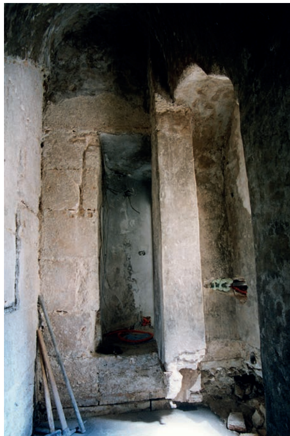
Fig. 11. Room beneath the Roman vault of the upper flight of the staircase north of the Palace's western gate (photo: K. Marasović)
