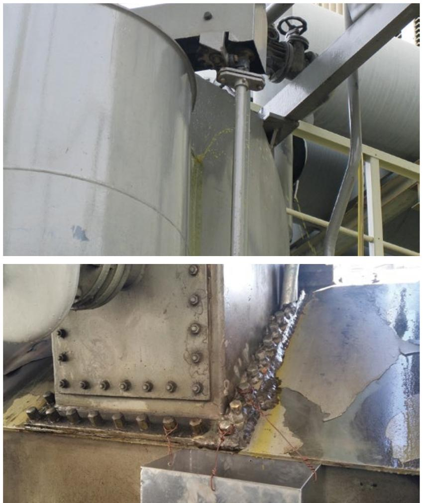
Figure 4. Leaking transformers need to be sealed
