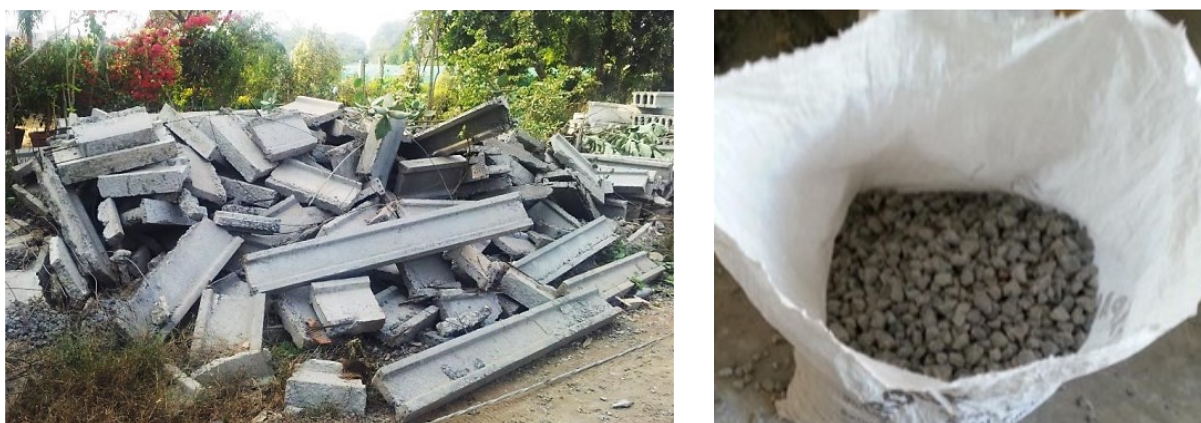
Figure 1. Production of recycled coarse aggregate from demolished waste
