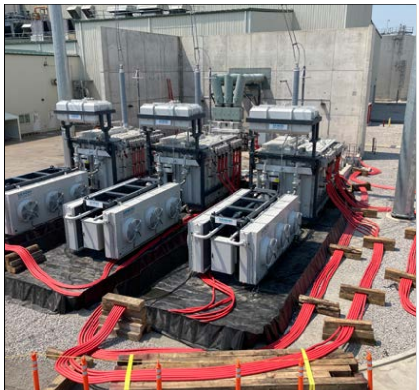
Figure 5. Site picture during Sensformer commissioning
