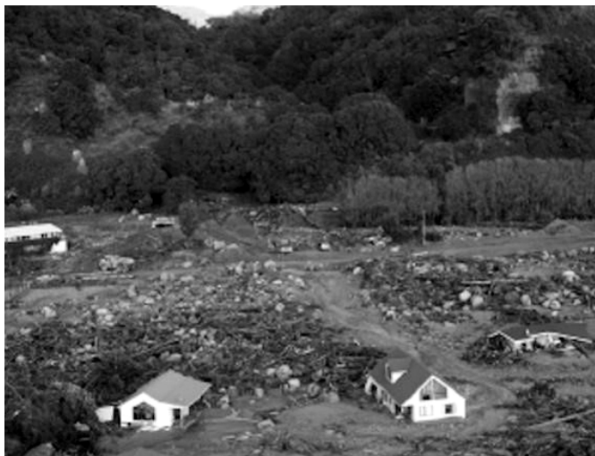
Figure 1. Debris and damaged houses following the 2005 Matatā debris flow (Source: Chappell 2013)
