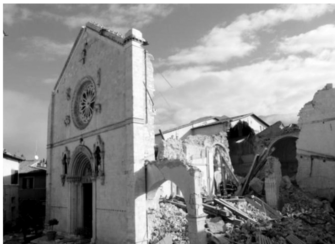
Figure 6. South wall and the facade of the Basilica in Norcia – after the earthquake in 2016. https://uss-sisma2016.beniculturali.it/interventi-sul-territorio/umbria/basilica-san-benedetto-norcia/ (Author: Ministry of Culture in Italy)
