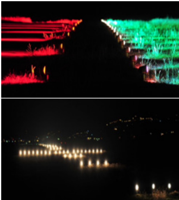
Figure 6 Airport Lighting System AP OMO, (intensity level III – end/threshold and approach light) [17]
