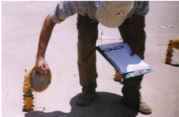
Figure 3 Confirmation of the sandblasting effect of the airport lights at the airports in Libya [13]
