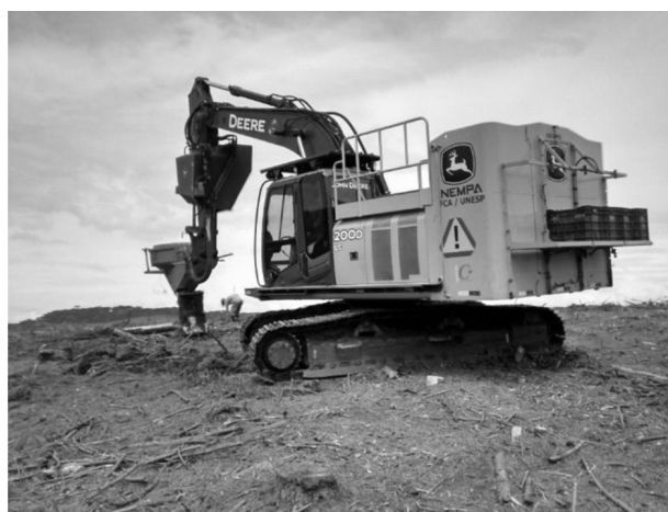
Fig. 1 Tree planter machine formed by a hydraulic excavator and mechanized planting equipment
