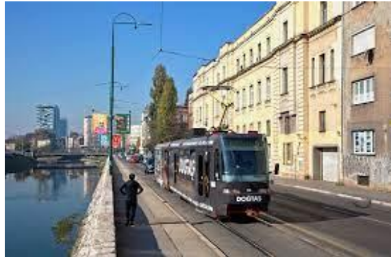
Figure 8. The bank protection for regulation of the right side of the Miljacka river and pavement curbs made of the Hreša limestone
