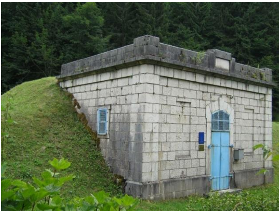
Figure 6. The tapping building at the Bistrica spring
