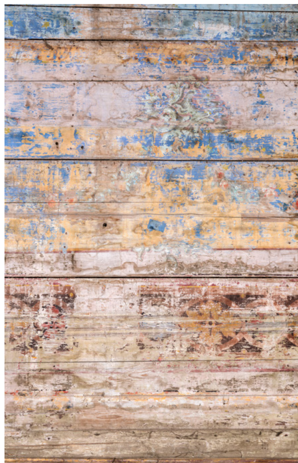
9. Detalj oslikane oplata svoda, kartuše s rokajima i girlandama te tragovima friza s geometrijskim motivima, zatečeno stanje (arhiva HRZ-a, snimka: G. Tomljenović, 2016.) Detail of the painted panelling of the vault, cartouches with rocaille decorations, garlands and traces of friezes with geometric motifs before conservation (HRZ Photo Archive, G. Tomljenović, 2016)
