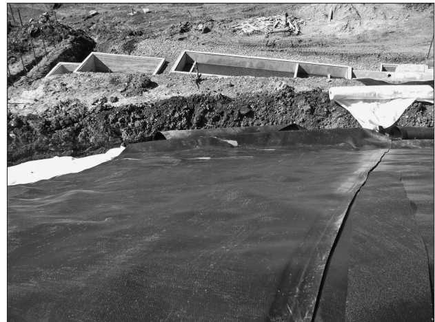
Figure 2. The ecological rehabilitation of a deposit with the use of geomembrane
