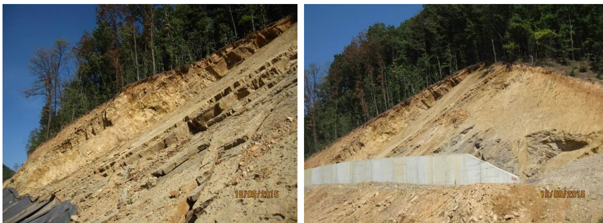
Figure 1. and 2. Planar sliding of rock blocks above a local road
