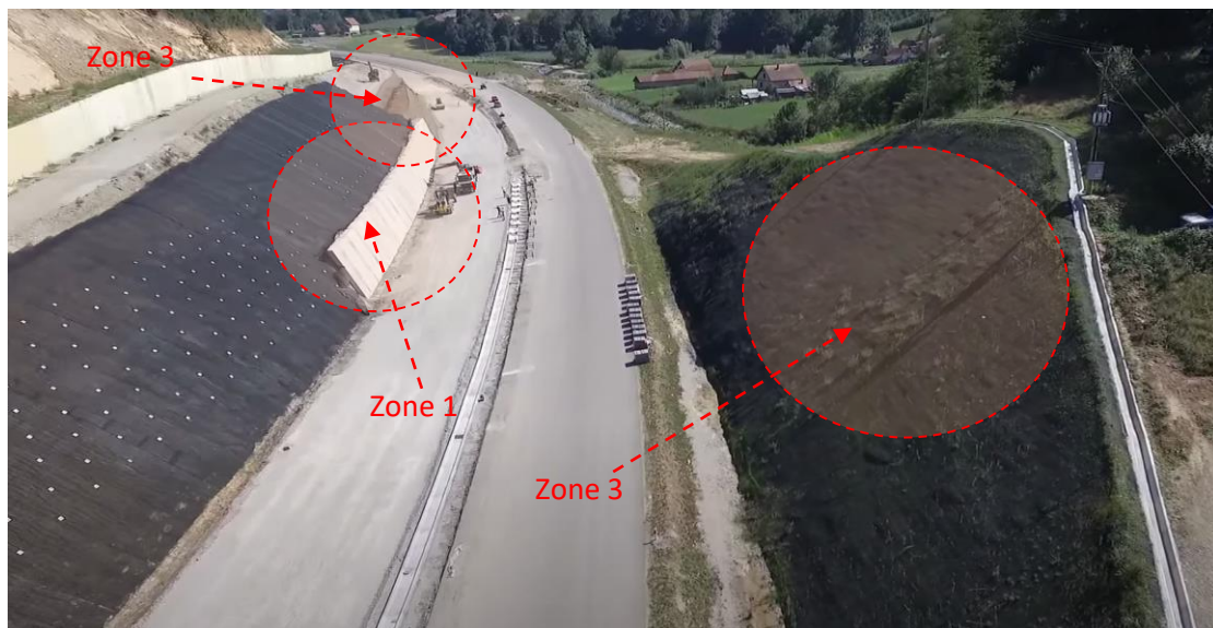
Figure 16. Left and right side of the cut after rehabilitation (with marked position of characteristic zones)
