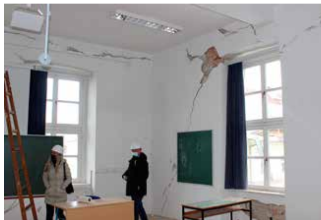
7 Petrinja, zgrada Srednje škole, inženjeri-konstruktori vanjski suradnici Ministarstva kulture i medija, Martina Vujasinović i Hrvoje Podnar u pregledu oštećenja i stanja zgrade (foto: T. Petrincec, MKM, 2021.) Petrinja, High School building, Ministry of Culture and Media associate structural engineers Martina Vujasinović and Hrvoje Podnar inspecting the damage and condition of the building (photo: T. Petrincec, Ministry of Culture and Media, 2021)
