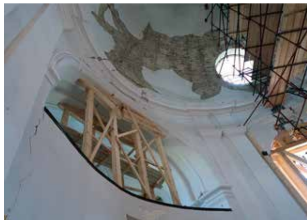
21 a b Opening of joints between the vault and the external walls of the skylight windows (photo: X. Romão, July 2021)
