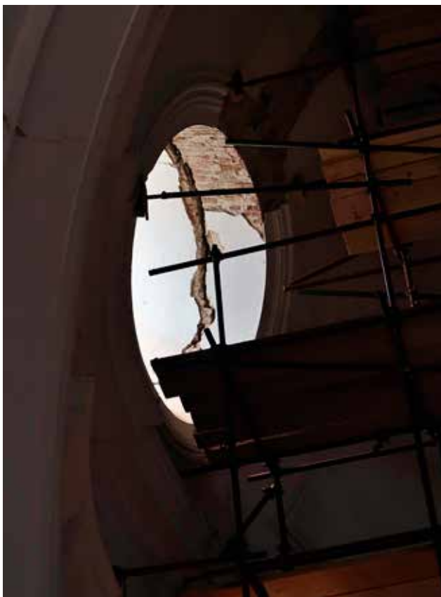
21 a b Opening of joints between the vault and the external walls of the skylight windows (photo: X. Romão, July 2021)
