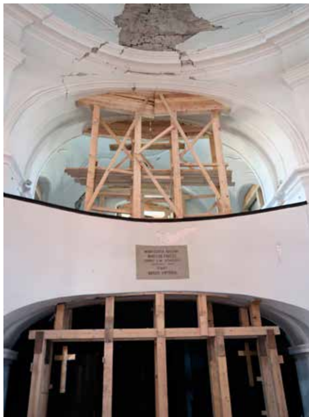
22 Shoring of the arch supporting the upper-choir, (photo: X. Romão, July 2021)
