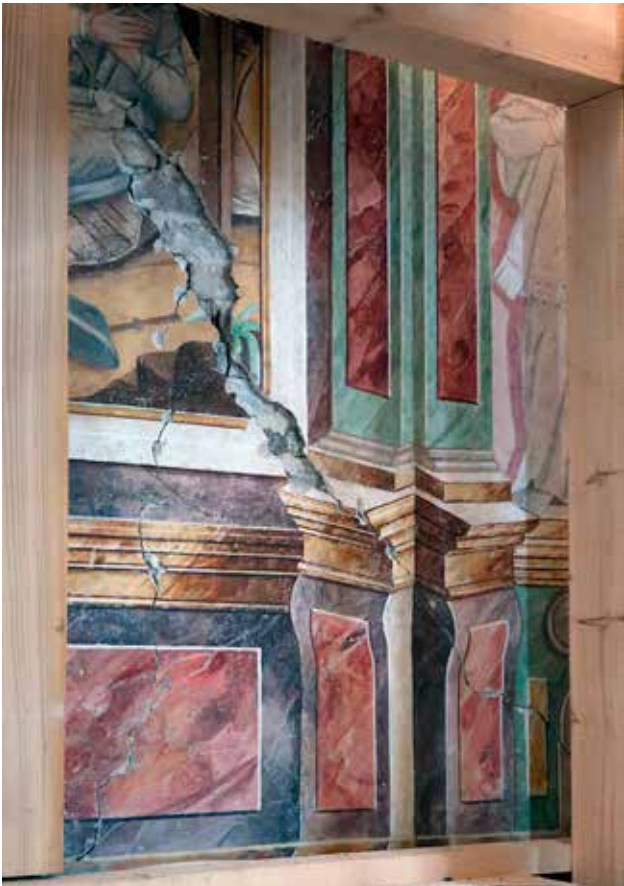
19 Missing parts of a mural painting in the lateral altars (photo: X. Romão, July 2021)
