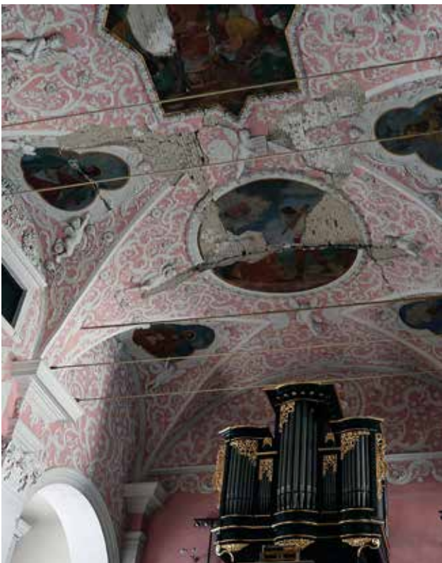
11 Detachment of finishing plasters of the nave vault (photo: X. Romão, July 2021)
