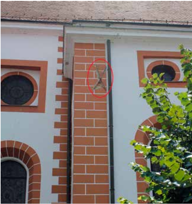
7 Anchorage points of one of the tie rods of the triumphal arch seen from the outside a) view of the left lateral wall where masonry crushing can be seen and, b) view of the right lateral wall where there are no signs of masonry crushing (photo: X. Romão, July 2021)
