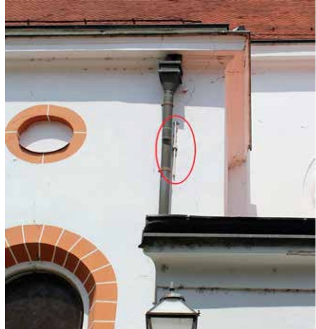
7 Anchorage points of one of the tie rods of the triumphal arch seen from the outside a) view of the left lateral wall where masonry crushing can be seen and, b) view of the right lateral wall where there are no signs of masonry crushing (photo: X. Romão, July 2021)
