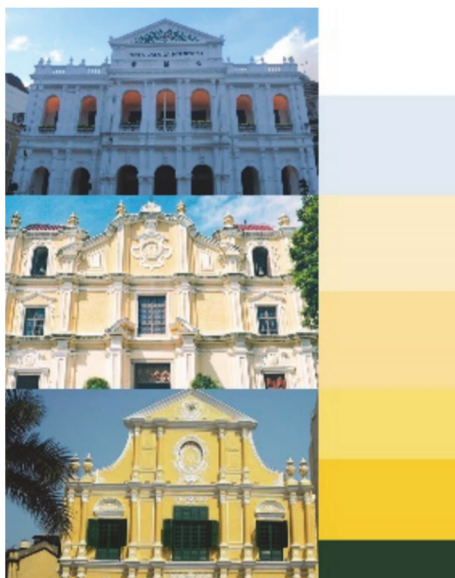
Figure 3 Building façade with light color tone
