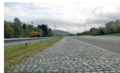
Fig. 6 Block pavement road
