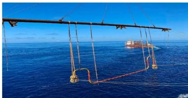
**Fig. 1** Typical M-type subsea jumper
