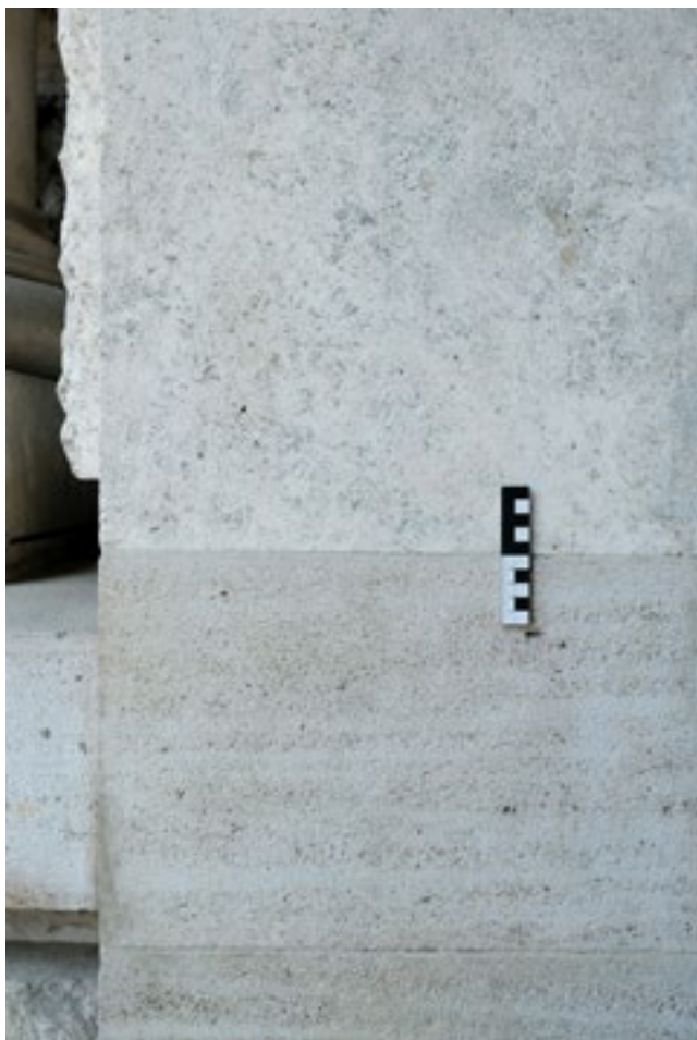
Fig. 8. Detail of door soffit–Wöllersdorfer at the lower part and Pula limestone at the upper, 2022
