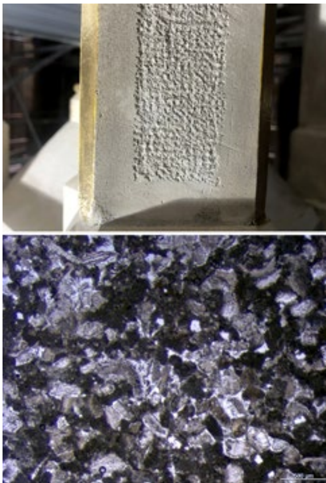
Fig. 3. Top: stone surfaces worked with a stock-hammer, 2021. Bottom: micrograph of the stone's texture (optical microscope, plane-polarized light, OM-PPL)
