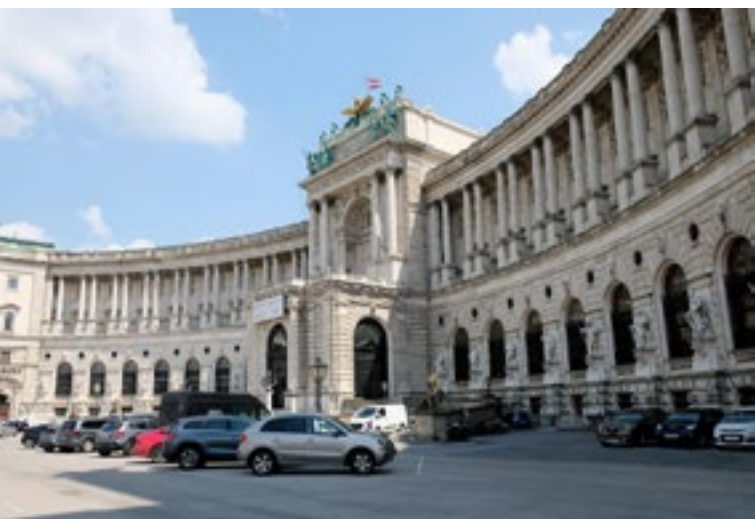
Fig. 16. Overview of the facade of the Hofburg, 2022
