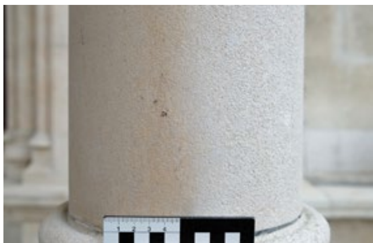
Fig. 4. Detail of a column at the loggia, 2022
